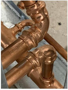
The Domestic Water System Design for this project required a Tee with the Branch leg larger than the Inlet or Outlet legs. This particular size is not standard in the fittings industry. This challenge was solved by using CerroPress Bushing Reducers to accomplish the engineer's design. (below)
